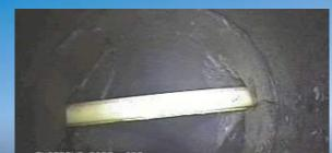
INCIDENT CODE: OBI INCIDENT DESCRIPTION: OBSTACLE - OBJECT PROTRUDING THRU WALL FEET: 0122.6 PERCENTAGE: 50 PISTITIN: 3 TO 9
