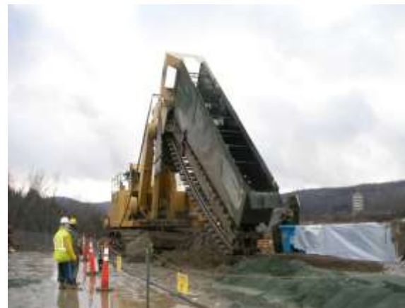
Photo: Dewind One-Pass Trenching
