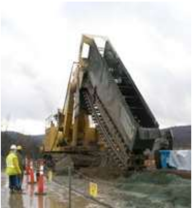
Photo: Dewind One-Pass Trenching
